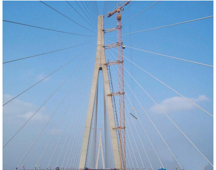
The bridge is located above the Yang Tse river near Nantong. It was constructed with 2 steel and concrete piles reaching 300 m high. The bridge has an overall span of 1200 m. Each pile was built by a MD 3600 tower crane anchored at 6 levels. It was equipped with 2 hoist winches and trolleys : one 20 t trolley for constant loads and one 80 t trolley for heavy loads.
