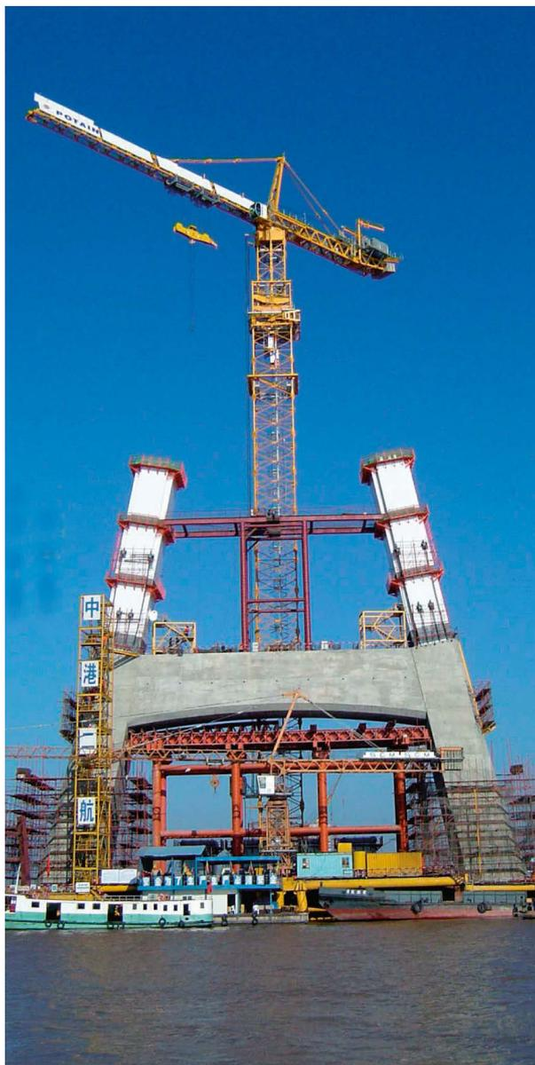
Two giant cranes MD 3600 participated to the construction of the the 3<sup>rd</sup> Nanjing bridge, located above the Yang Tse River. They were specially designed to lift steel structure elements of 160 t, used for the construction of the bridge piles.
