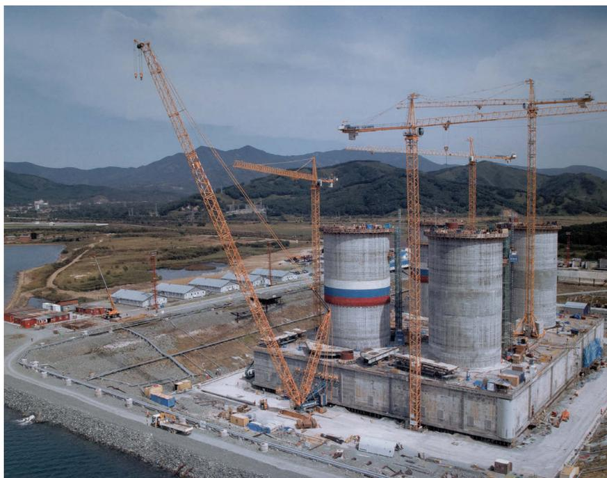
This project consists in the construction of an off shore platform in a drydock near Vladivostok (Eastern Russia). The yard is equipped with 5 cranes : 1 MDT 218 on a travelling chassis, 3 MD 485 B on fixing angles and 1 MD 485 B on chassis.
