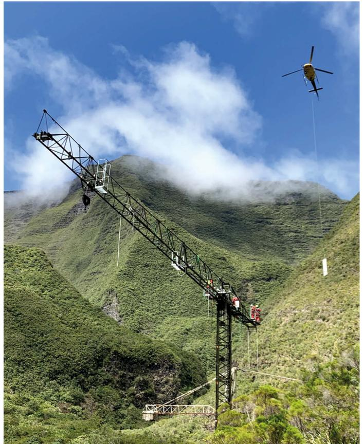
After manufacturing, the crane was shipped to the GLI yard on La Réunion, where the erection team practiced assembling and disassembling prior to installing it, to be sure of the weight, slinging points and work plan.
