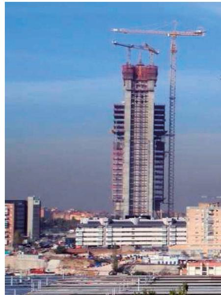
The Spanish company REPSOL ordered one MD 1400 and two MDT 302 for the construction of the «REPSOL TOWER» in Madrid. MD 1400 was erected up to 277,3 m with 7 anchorings and was used to lift 36 t at 38 m radius at 250 m height. Additional 20 t steel structures were installed on the top.
