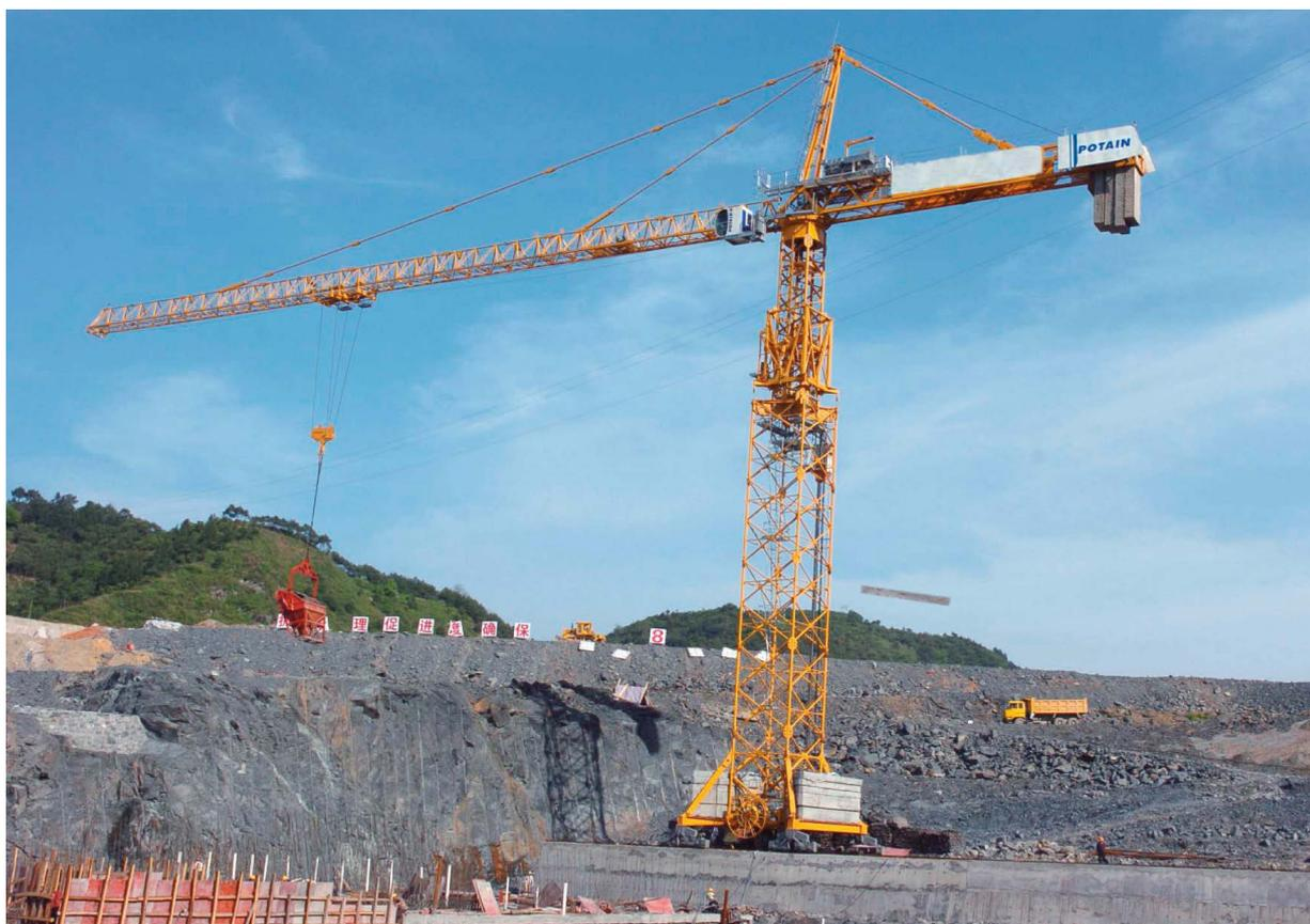
The Qingshuitang Dam is located in the Hunan Province - China, 72 km from Huaihua city. Gezhouba corporation acquired 2 units of MD 1100 (40 t capacity version) for the dam concreting. Both cranes operate with 6 m<sup>3</sup> bucket (20 t) up to 52 m radius (jib 70 m) and 3 m<sup>3</sup> bucket (10 t) from 52 m to 80 m radius.
