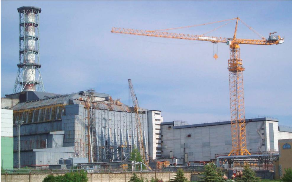
The MD 3200 was used to reinforce the collapsed nuclear power plant before complete recovery with the new shelter «sarcophage».
