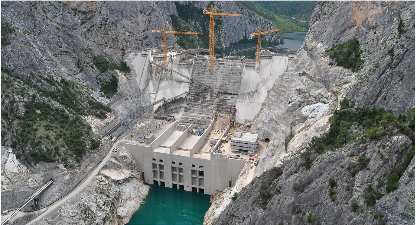
The Boyabat dam project was made with conventional vibrated concrete (CVC), built by blocks using conveyor system and tower cranes. It is located in North Central Turkey near the Black Sea. The main purpose of the tower cranes is to handle 20 t loads such as reinforcement, rebars, conveyor trusses, penstocks and 9 or 6 m<sup>3</sup> of concrete buckets anywhere on the dam project.
