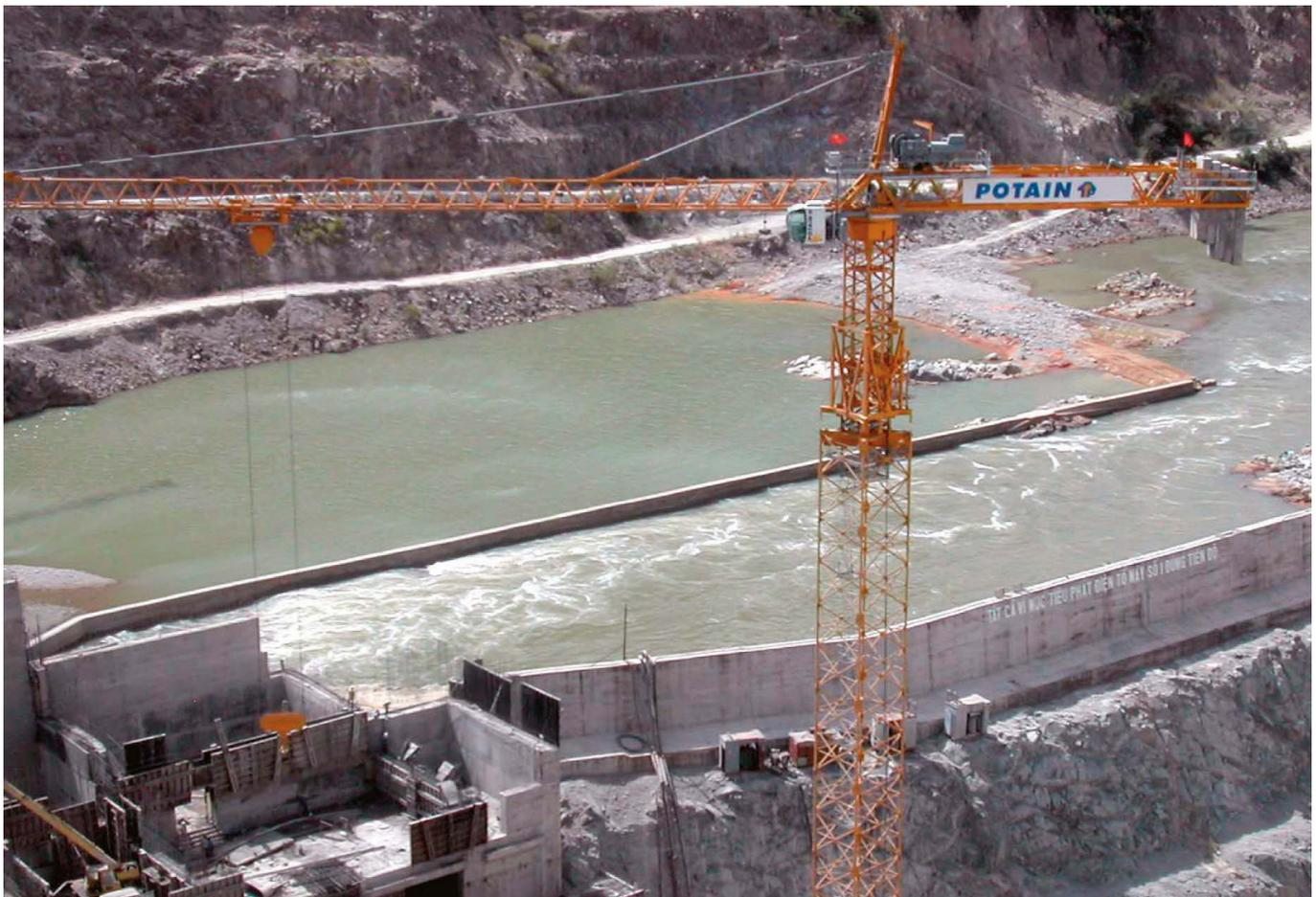
The Vietnamese Son Da Corporation company ordered 4 MD 900 B cranes for dam construction. The 250 LCC hoisting mechanism enables a productivity of approx. 70-80 m<sup>3</sup>/h depending on the site conditions. Trolleying and slewing mechanisms with frequency variations.
