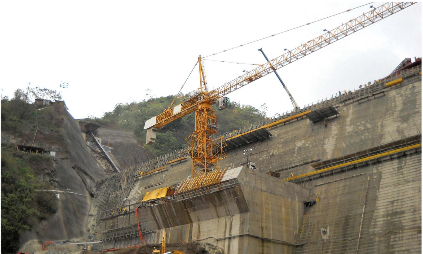
Pirris is one of the largest dams ever built in Costa Rica. ICE company purchased a new MD 1100 to build the dam. The crane has been chosen for its outstanding performance and its compactness for transportation. Considering the seismic constraints of the jobsite location, the crane was reinforced to withstand maximum accelerations of 0,16 g.
